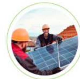
Decarbonisation of heating and cooling
