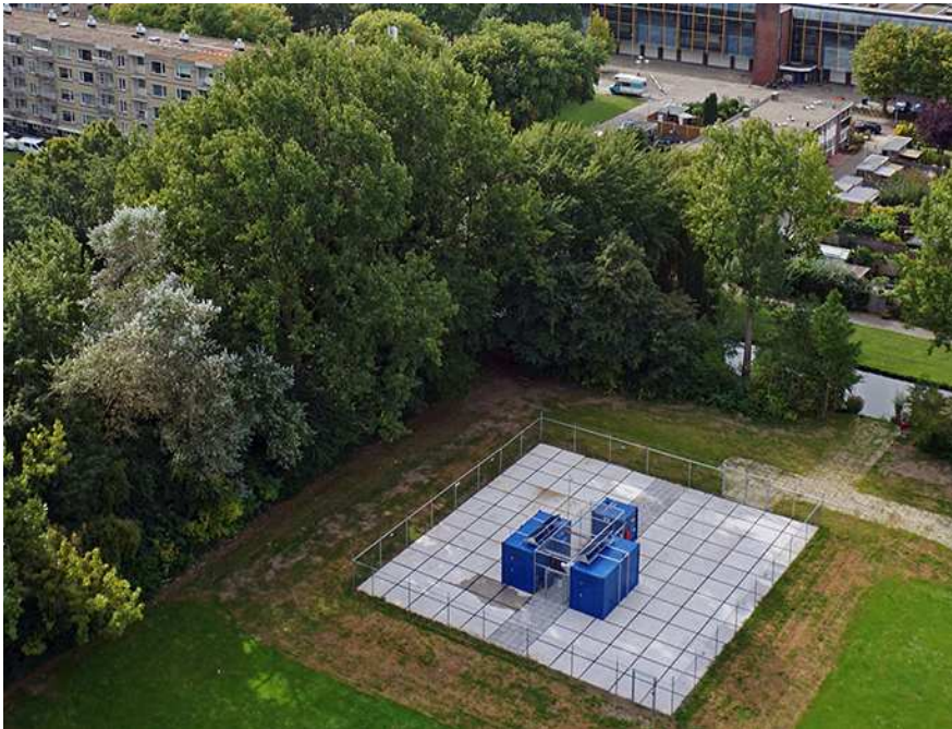
Green hydrogen production
